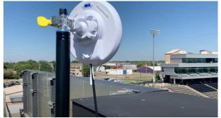
\*Be sure the antenna has a clear and straight line of sight to the press box antenna
